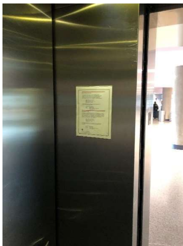
Landside A Elevator
