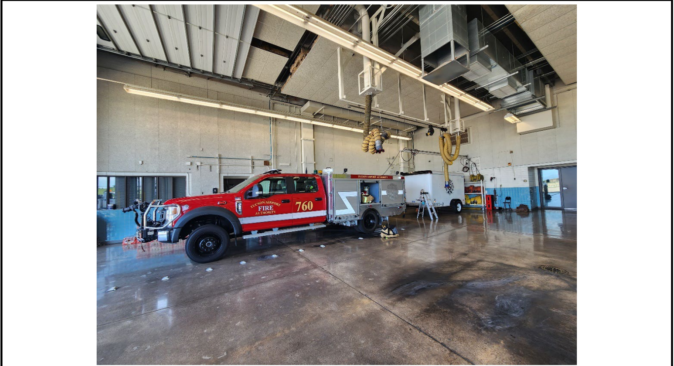
Location/Description: AOC 29: Current TAA Fire Station (B-284)
