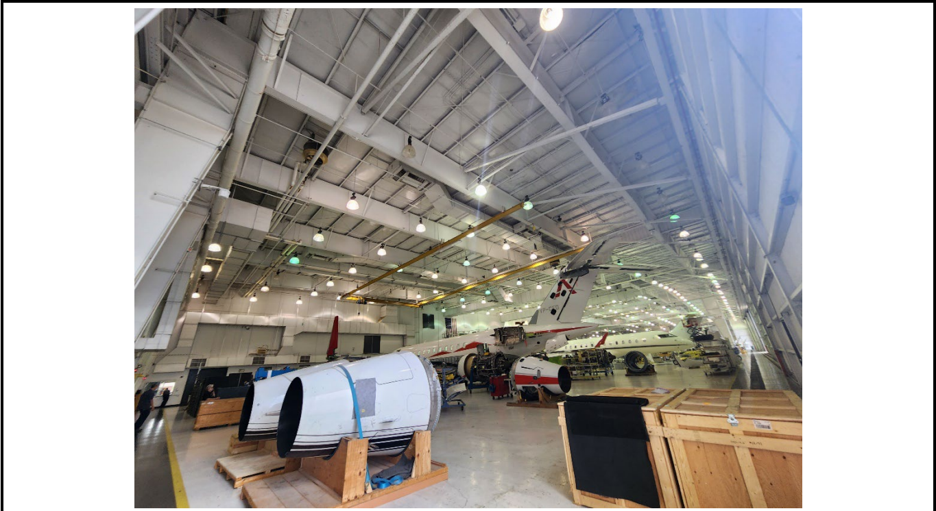
Location/Description: AOC 24: Bombardier Building S – view of hangar
