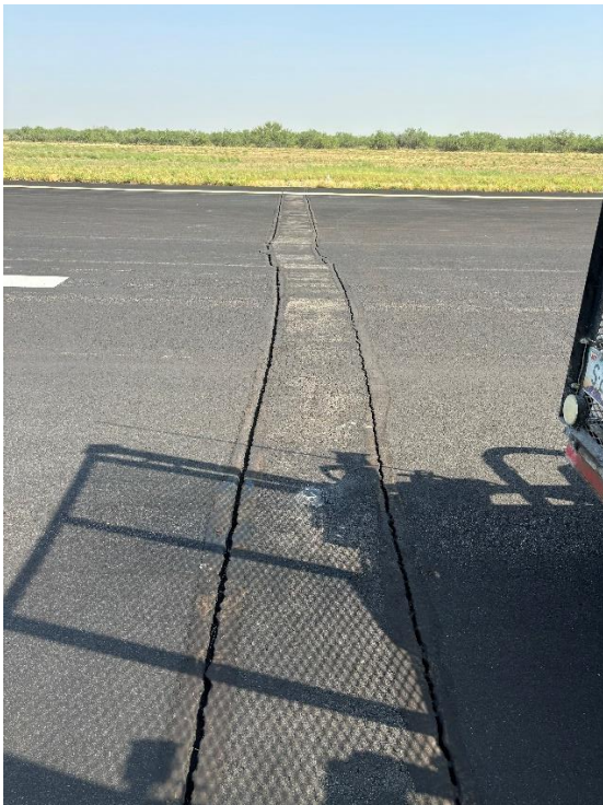
R2. View north.
