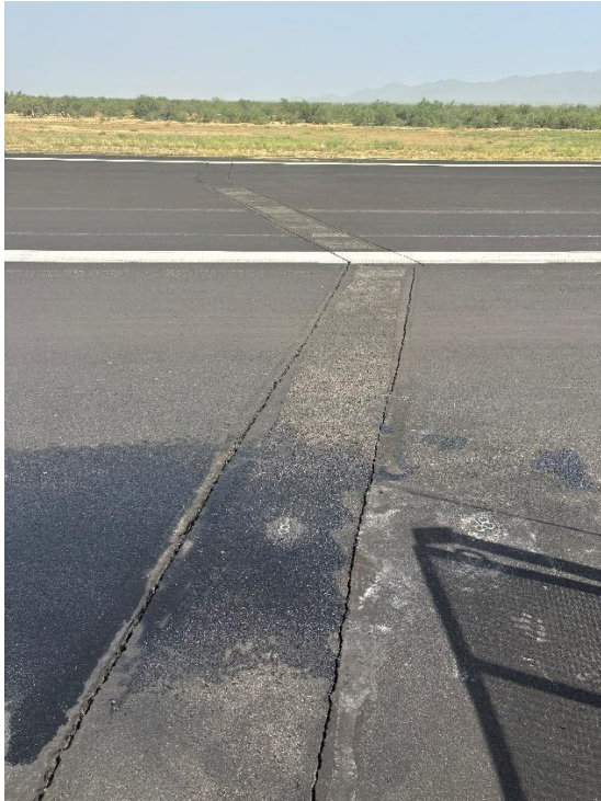
R7. View north.
