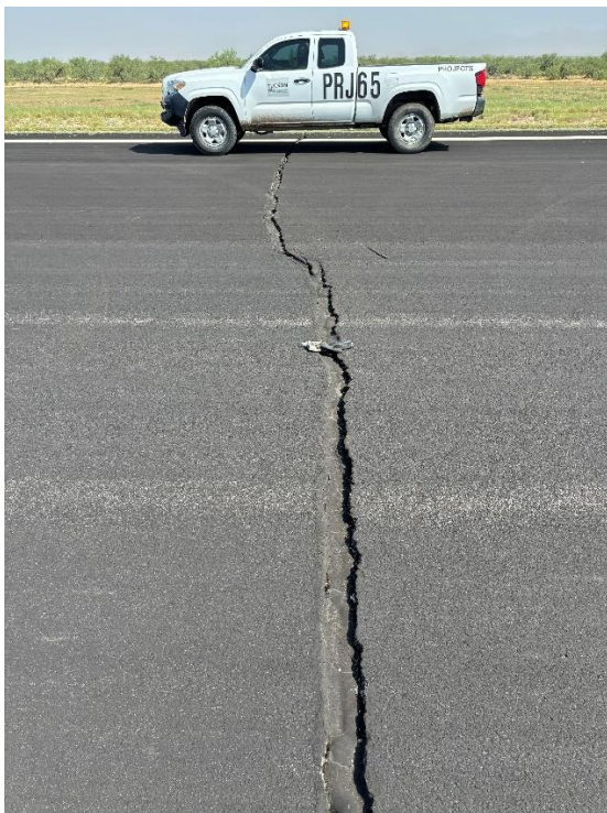
U2. View north.
