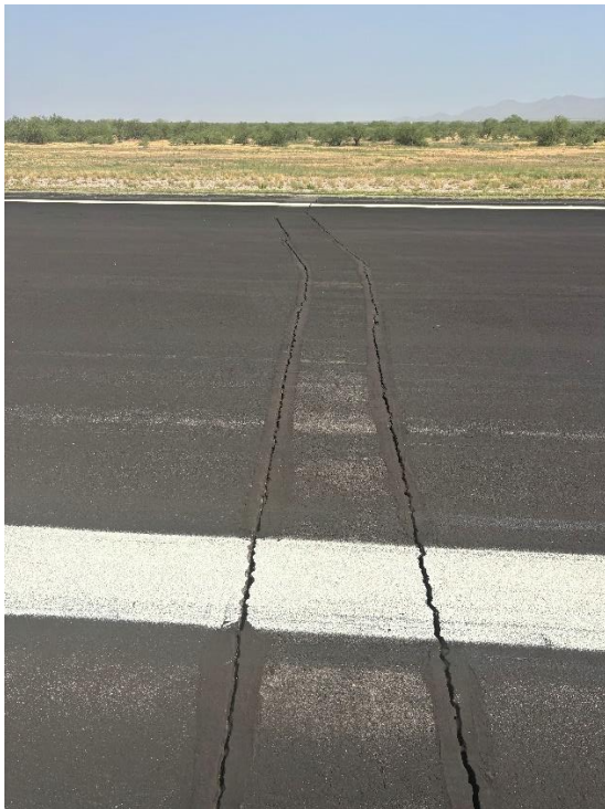
R8. View north.
