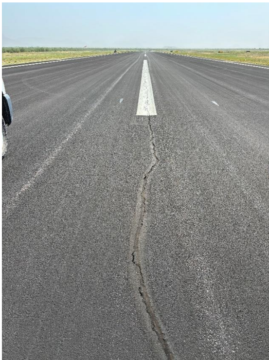
L1. View west.
