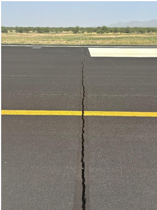
U4. View north.
