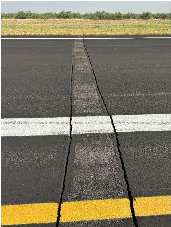
R4. View north.
