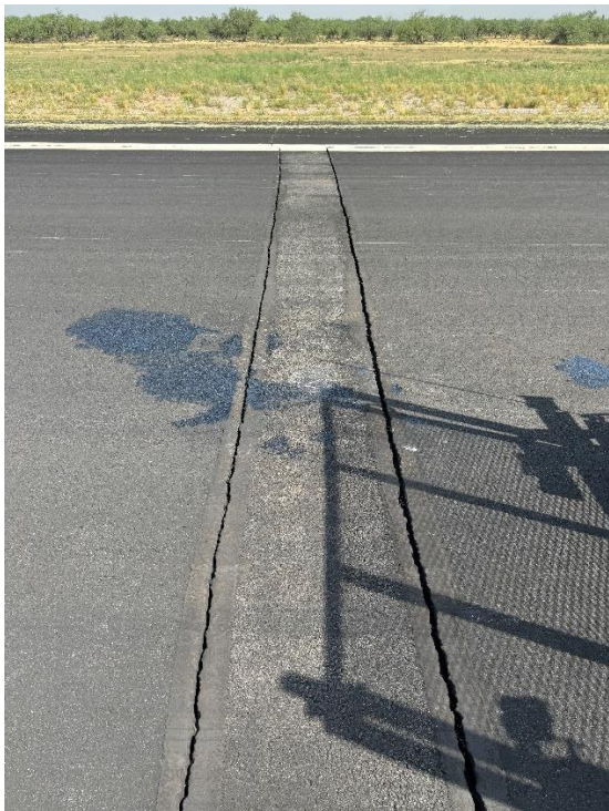
R6. View north.
