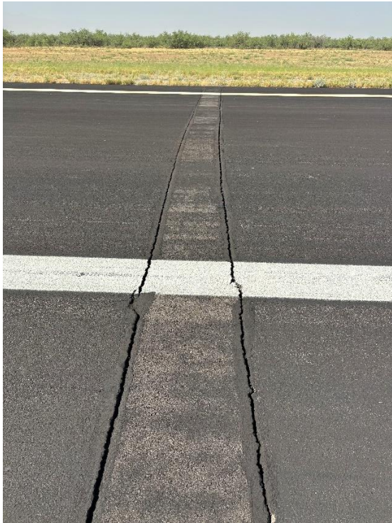
R3. View north.
