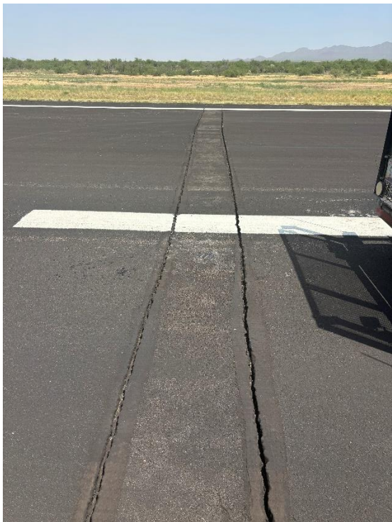
R10. View north.
