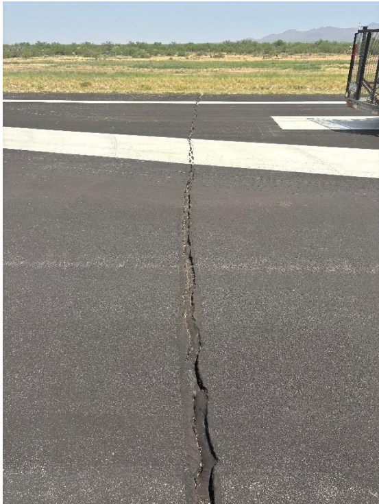
U5. View north.
