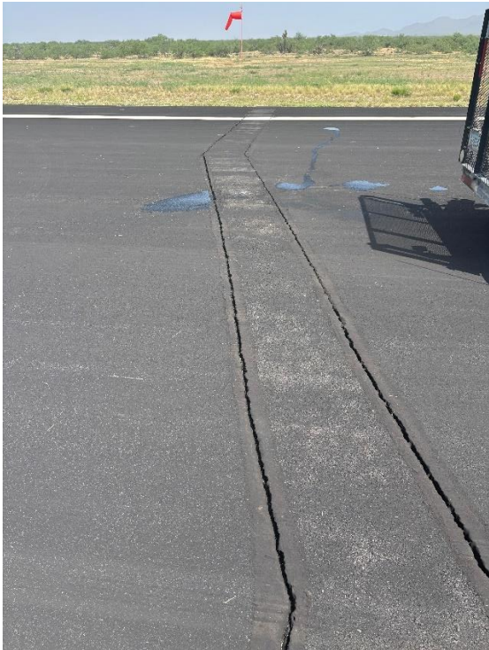
R9. View north.
