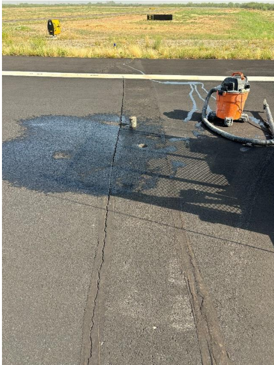
R1. View north.
