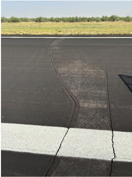
R5. View north.
