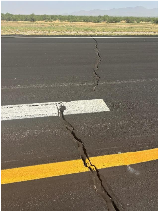
U3. View north.
