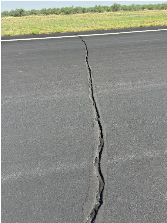
U1. View north.
